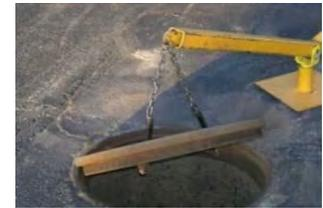
Visually inspect all chambers for heavy sediment, trash and debris loading. A battery powered flashlight or droplight is recommended for thorough inspection.
