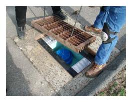
Both the StormBasin and StormSack are designed to be installed beneath the iron storm sewer grate capturing the water as it flows off the surrounding surfaces. In this position the grate and the StormBasin or StormSack share the same mounting ledges.
