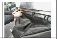
The StormSack is now complete with new filter bag attached. Repeat the process for Double unit storm sewer inlets
