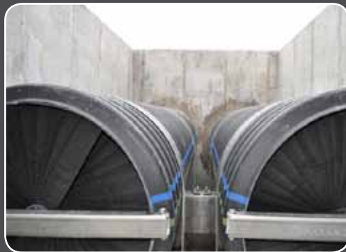
30" diameter corrugated plastic pipe houses filter elements
